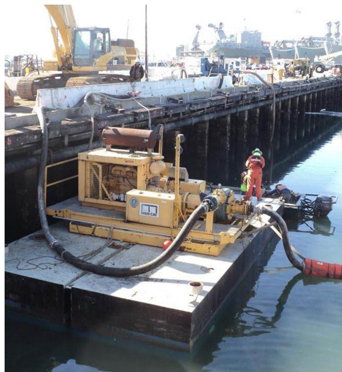
Dredging at the Wharf
