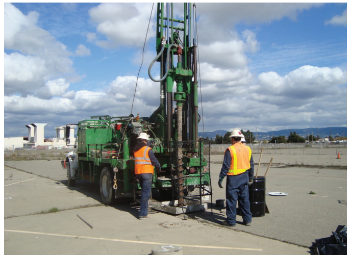
Dual Vacuum Extraction Well Installation at Building 410
