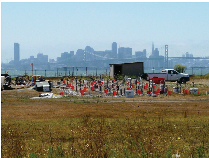
Site 1 Chemical Oxidation Treatment
