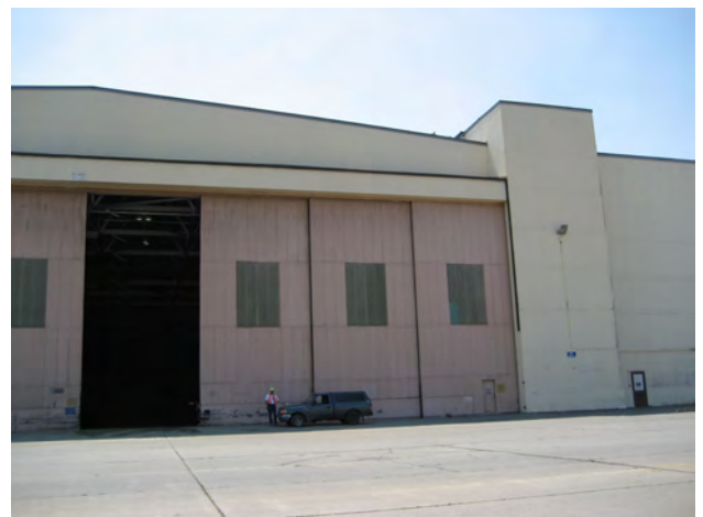
12. View of the exterior wall structure on Building 5A. Note the concrete and painted steel beams within the wall.
